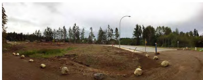
The opportune time to retain native soils is following land clearing and prior to soil compaction practices.
